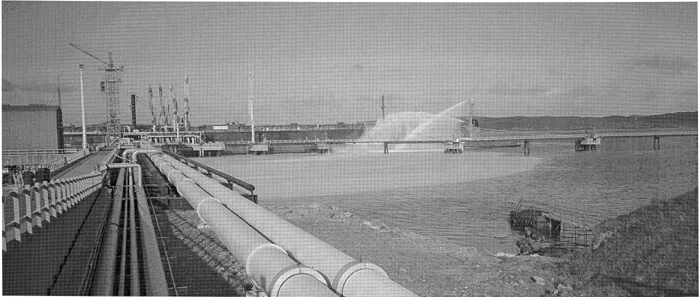
Fig. 2. Fire-fighting foam deployed for oil-spill simulation at Sullom Voe oil terminal (1988).
